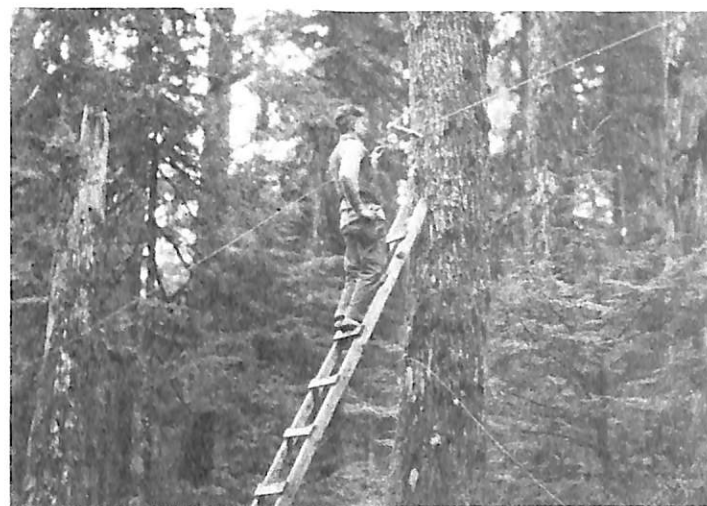
Figure 9. Wooden bracket for Forest Service field telephone lines, designed by Clay M. Allen, Pacific Northwest District (now Region) telephone engineer, to hold the wire away from the trees and thus prevent leakage of current, which would be extensive in the wet weather so common on the west side of the Cascade Mountains in that Region. 1921 photo. (NA:95G-158323)
