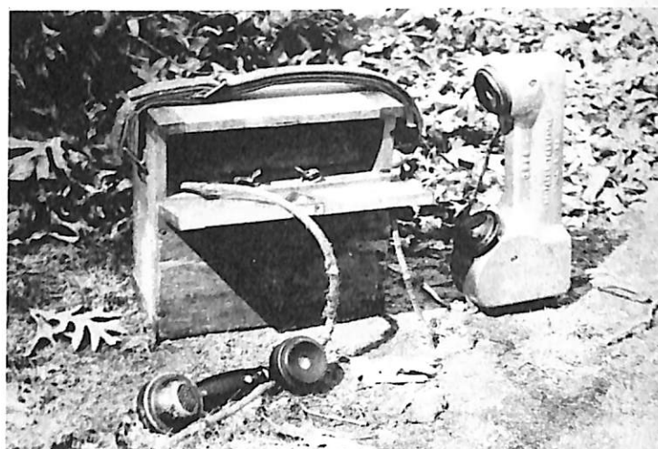
Figure 111. A strong emphasis on portability in communications began early on the National Forests. These Forest Service portable telephone handsets, made by Kellogg, were carried by Rangers and clamped to field telephone lines for use. Wooden box model (C-608) has a folding crank on the right side. The front is hinged to open down. This model, which dates from the late 1920's, was used through the 1930's. A more truly portable set in the modern sense, the aluminum model B-209 dates from the late 1930's and was used through the 1940's. It has an external contact for the telephone wire and two buttons to press--one to send a sound to alert the other party on the line, and one to press while talking. (Forest Service photo, History Section)
