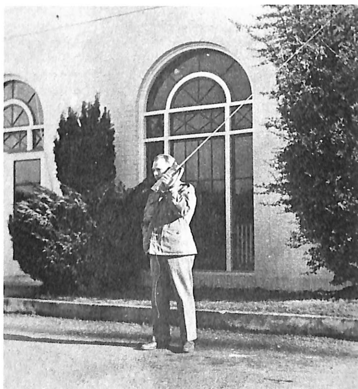
Figure 126. Type SF handie-talkie being demonstrated at the Radio Laboratory by Logan Belleville. (Forest Service photo, History Section)
