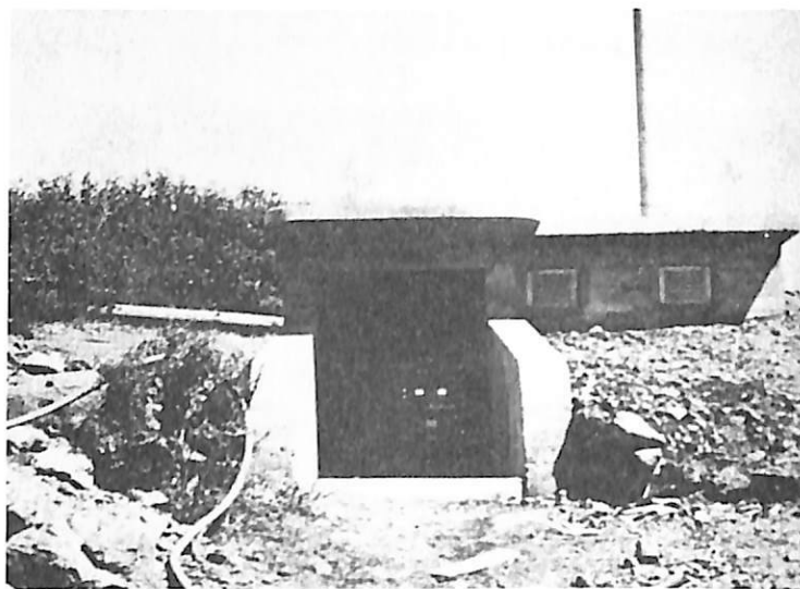
Figure 77. The RRS (Radio Relay Station) installation atop Mt. Diablo, Calif., first field setup of the Forest Service, July 1941. It allowed the nearby Regional headquarters in San Francisco to establish point-to-point communication with any outlying vhf radio within visible range of the repeater. Esthetics required the RRS to be placed in a plain building that minimized environmental impact. (Forest Service photo, History Section)
