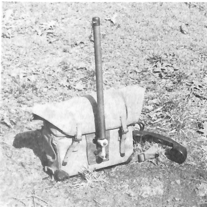
Figure 130. An early Link lightweight FM radiophone packset (model 695-B). It was purchased in the early 1950's by the Forest Service under competitive bid on the basis of specifications developed by the Radio Laboratory. (Forest Service photo, History Section)
