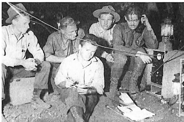
Figure 97. Message center at night on the Barley Flats fire, Angeles National Forest, southern California, December 1936. Shown is the TH/TL set with separate circuits on the 10-meter band for reception and transmission, described in chapter 7. See figure 72. (NA:95G-341687)
