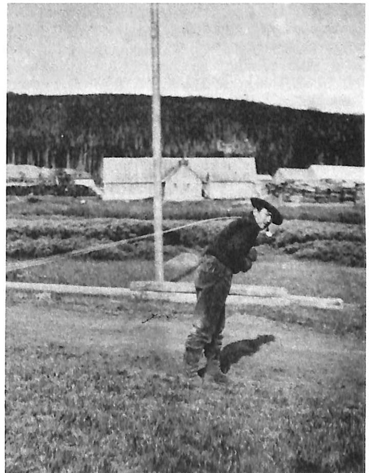
Figure 2. Ranger stringing telephone wire and setting poles on the Big Horn Forest Reserve, northern Wyoming, August 1906, for the first Forest Service telephone line, 109 miles long. (National Archives: Record Group 95G-69555)
