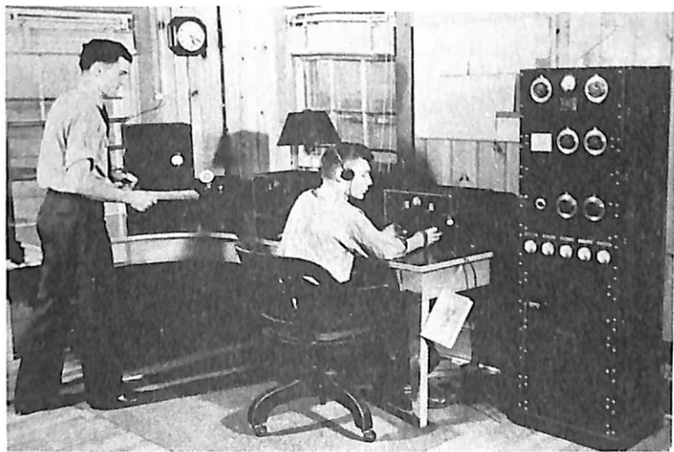
Figure 113. Allen Thompson and Jeffrey Geiser, right, operating KBCX, the Northern Region control station at Missoula, Mont., in 1937. William Apgar's powerful "home-brew" transmitter is the floor model unit at far right. The Region was ordered by the Washington Office to reduce its power in January 1941. (Forest Service photo, History Section)
