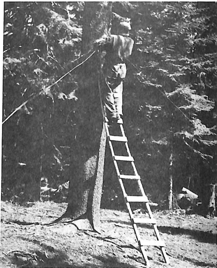
Figure 118. Civilian Conservation Corps (CCC) enrollee installing a single-wire, ground-return telephone tree line on the Columbia (now Gifford Pinchot) National Forest, Wash., in 1939. (NA:95G-380399)
