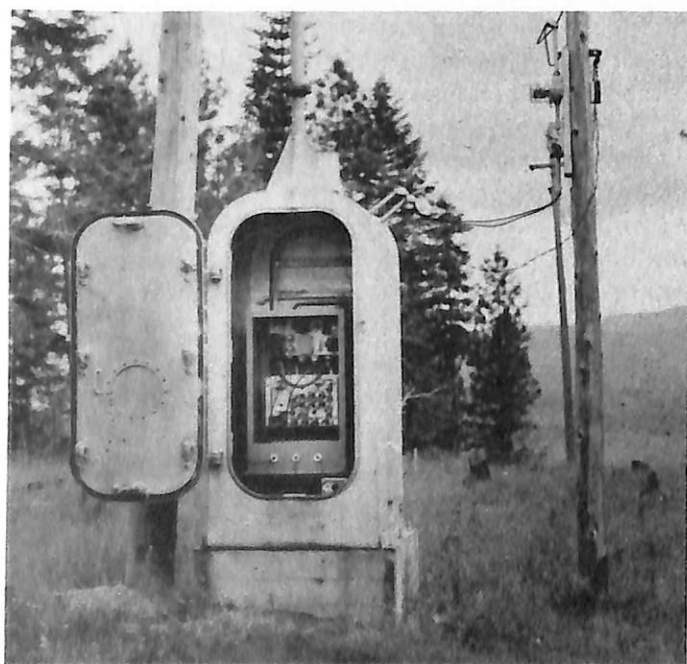
Figure 119. Unmanned Forest Service radio relay repeater stations at remote sites, housed incongruously but adequately in Navy surplus bulkhead, left, and in a former outhouse, right. These
