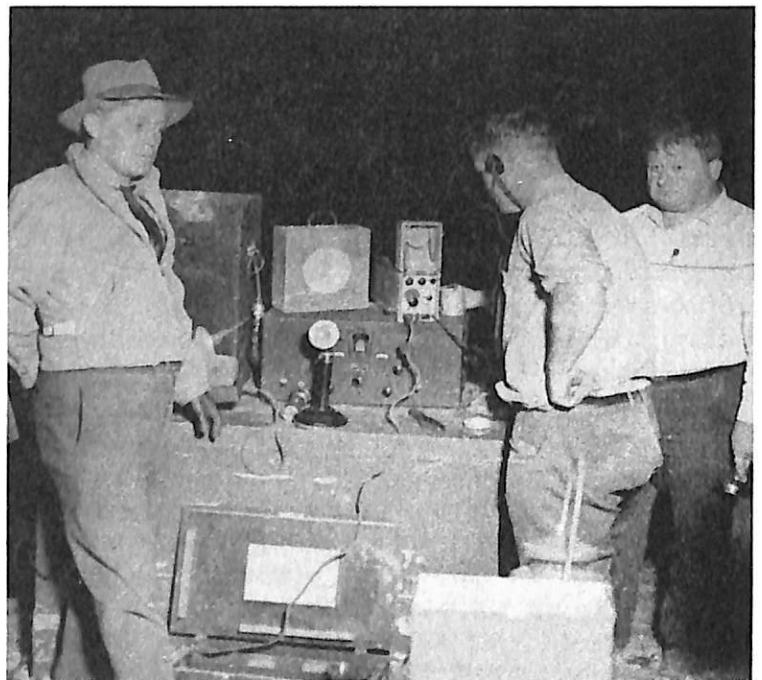
Figure 46. The Forest Service's small type PF set with speaker is on top of a Hammarlund Comet Pro commercial receiver in this photo. The receiver was used in conjunction with the Forest Service type M radiophone transmitter, which is visible behind Forest Supervisor William V. Mendenhall at left. This night photo was taken at the radio center on the Barley Flats fire, Angeles National Forest, southern California, in 1936. (NA:95G-341689)
