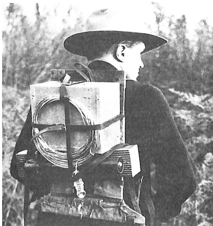
Figure 50. Portability of the type P radio is demonstrated by Harold Lawson of the Radio Laboratory. Note antenna loading coil and battery under container. (Forest Service photo, History Section)
