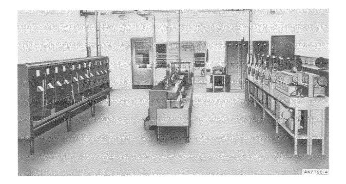
Teletypewriter Central Office Set AN/TGC-4 is a large semiautomatic tape relay facility for handling a large volume of teletypewriter traffic in fixed station applications. It must be specifically engineered and arranged for the traffic-handling requirements of the headquarters in which it is used.
